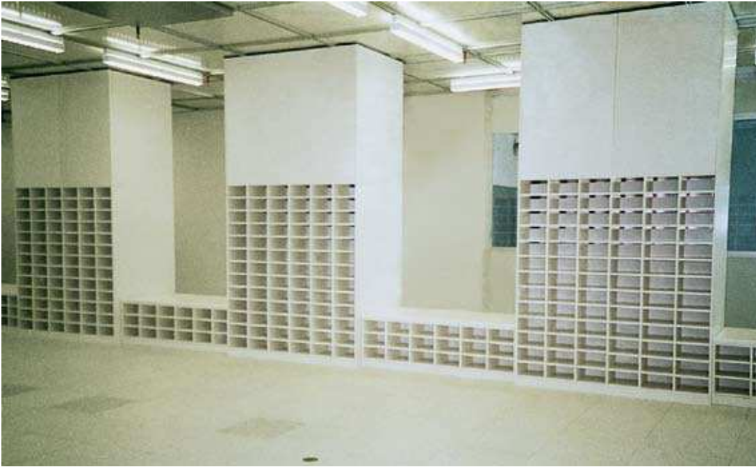
Gowning area with exhausting Sitover and shoe compartments in HPL Quality
